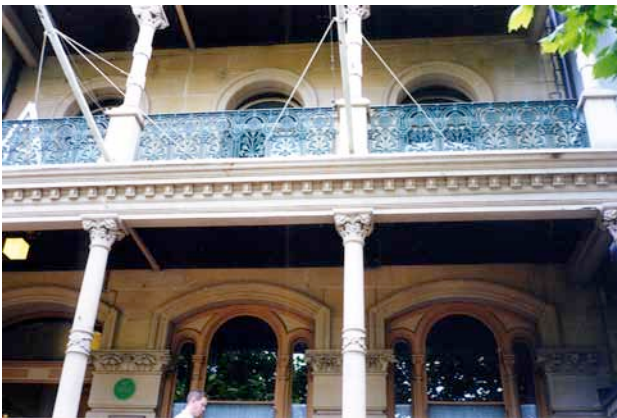
FIGURE 2.23: Verandah – First and second floors, looking north-west
