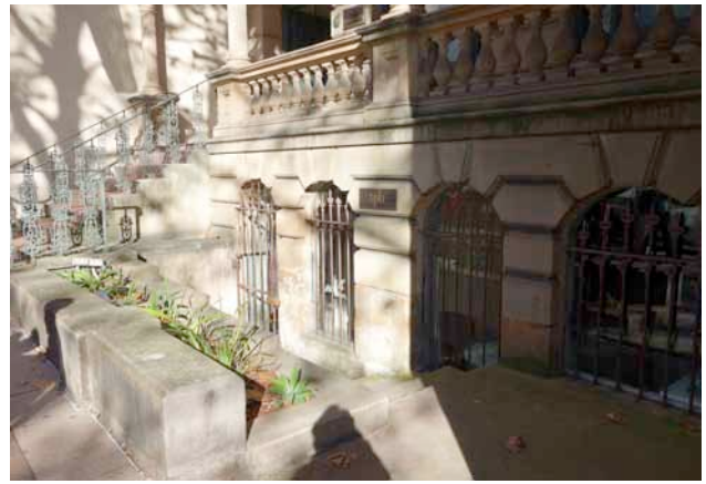
FIGURE 2.22: Basement façade and ground floor verandah
