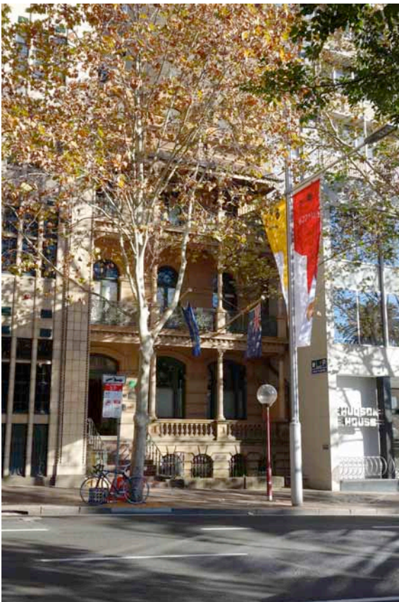
FIGURE 2.11: View C: filtered views looking north west from Macquarie Street.
