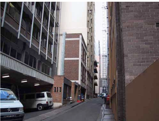
FIGURE 2.19: Phillip Lane looking south. History House is the 3-storeyed concrete-framed structure in the centre.
