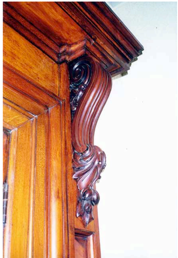
FIGURE 2.45: Detail of corbel to doorcase
