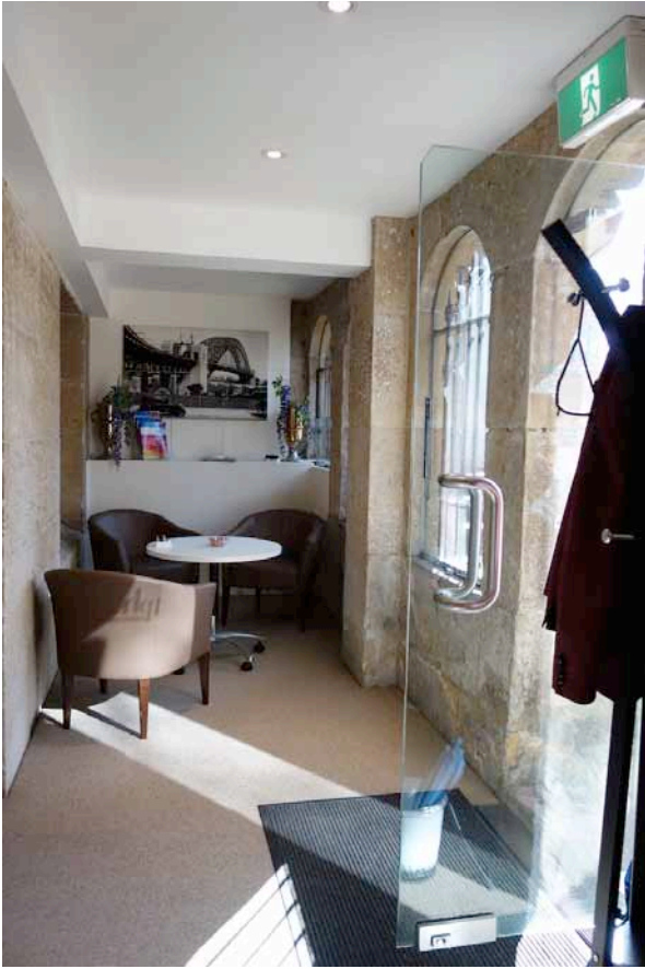
FIGURE 2.31: Basement entry located directly below the verandah, There is evidence of
