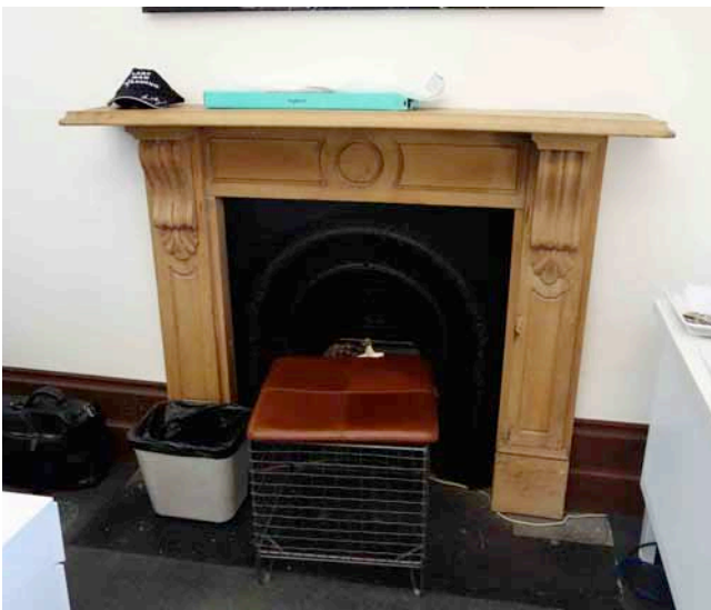
FIGURE 2.55: Late Victorian timber chimney piece (later insertion)
