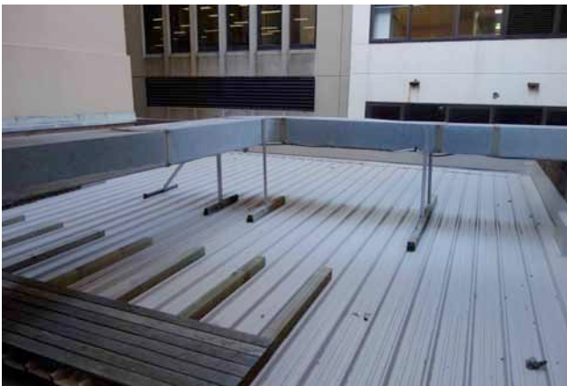
FIGURE 2.65: Roof over 1970's wing
