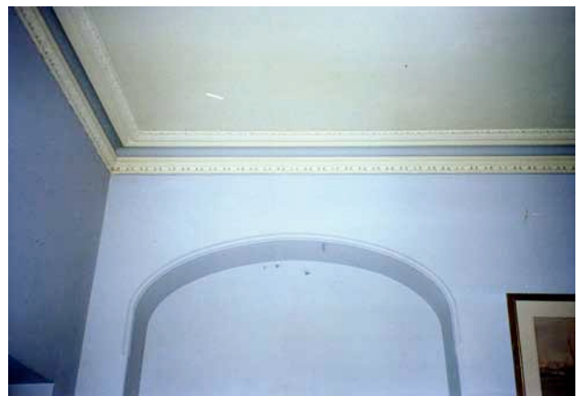
FIGURE 2.50: Original arched recess and cornice of north wall, first floor, centre room
