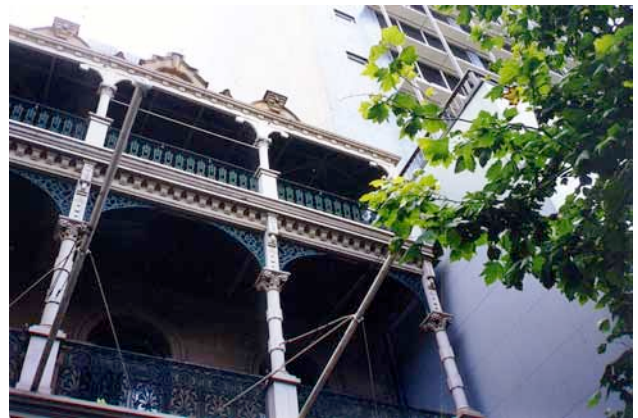
FIGURE 2.24: Verandah – ground and first floors, looking west
