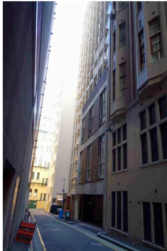
FIGURE 2.16: View H: Looking north along Phillip Lane. This view is terminated by the historic Chief Secretary's Building.
