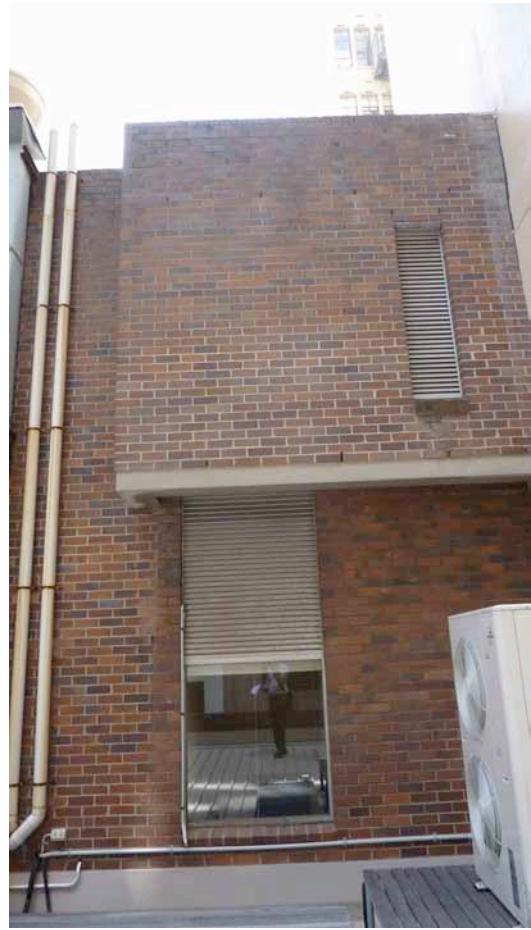
FIGURE 2.64: Rear of kitchen and fire stair wing at attic level
