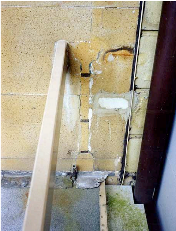
FIGURE 2.29: First floor verandah, evidence of north panel and louvered screen
