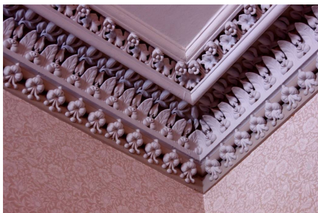
Figure 3.3.1 Reception Rooms, Moulded Plasterwork
